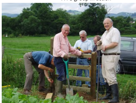
Installing a stile
