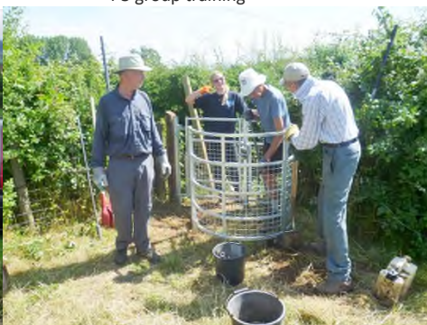
Installing a kissing gate
