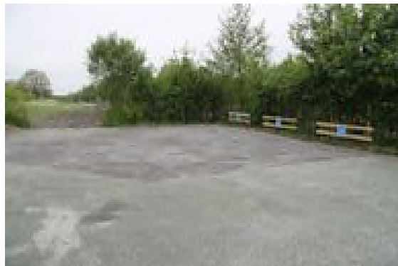
Completed car park
