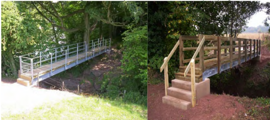
Two bridges installed by contractors under the capital programme
