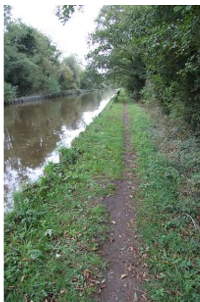
Towpath before work
