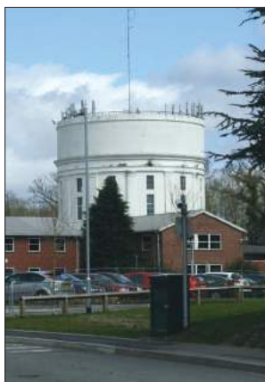
Water Tower of Severn Trent Water works.
