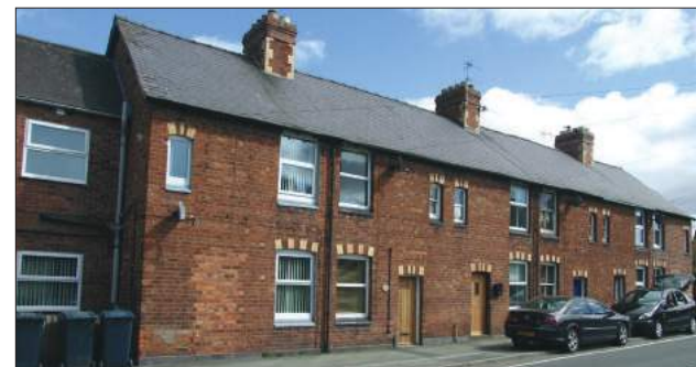
Terrace of Victorian houses on Welshpool Road.
