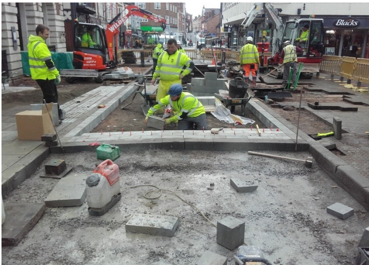
Commencing installation of yorkstone setts to pedestrian crossing in Shoplatch
