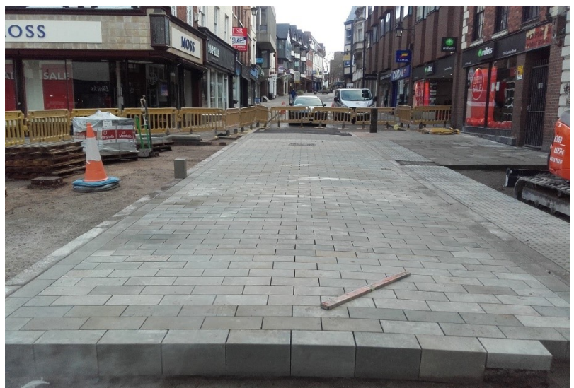
Pedestrian crossing with setts laid prior to grouting
