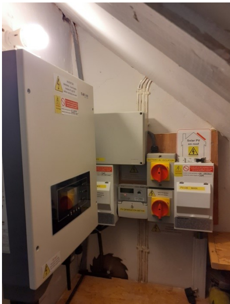
Sofar inverter / distribution box and Pylontech batteries in under stairs electricity cupboard
