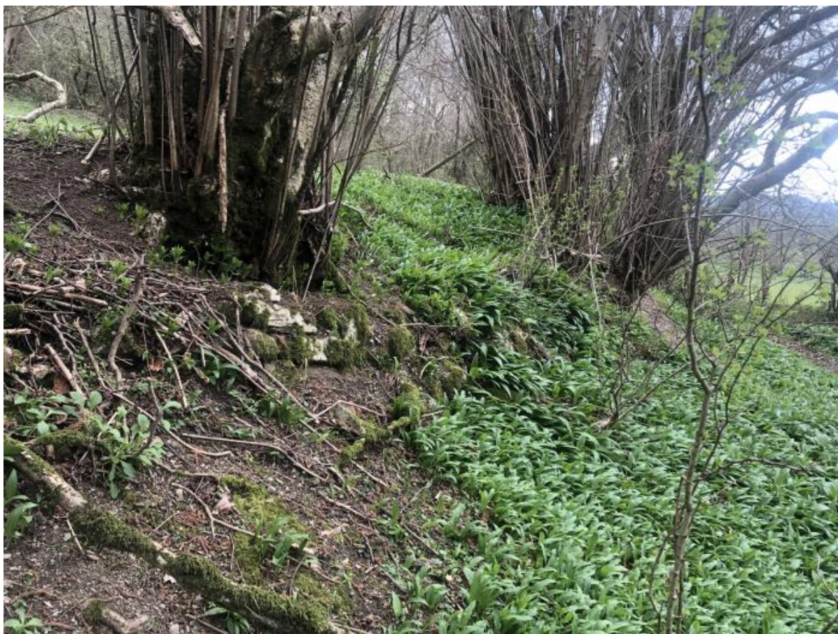
A possible build up of debris can be seen sloping from the retaining stones. It is covered with wild garlic and a couple of hazel saplings.
