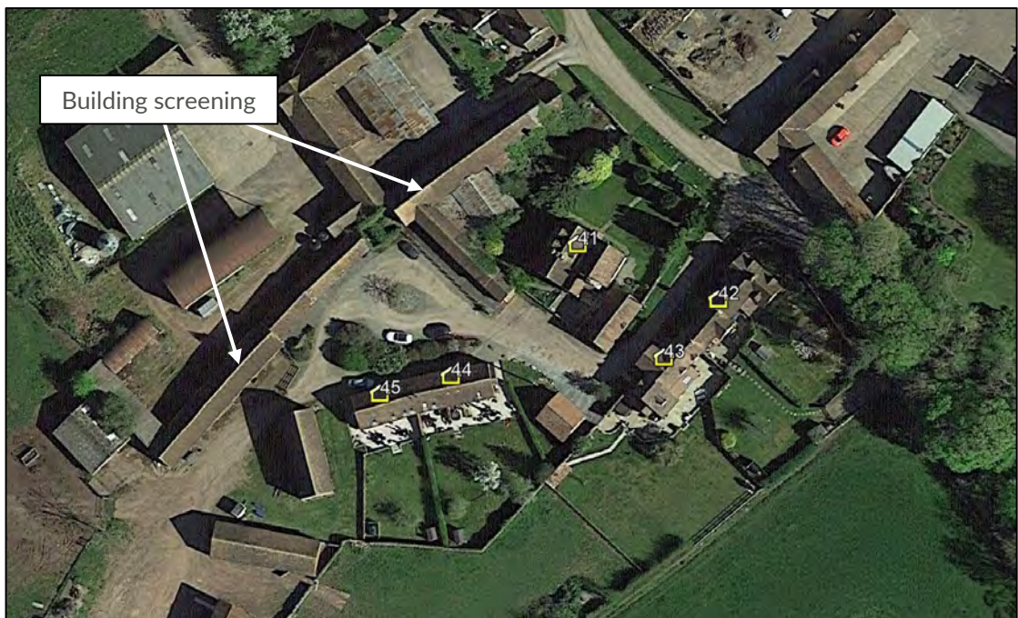
Figure 32 Building screening - dwellings 41 to 45
