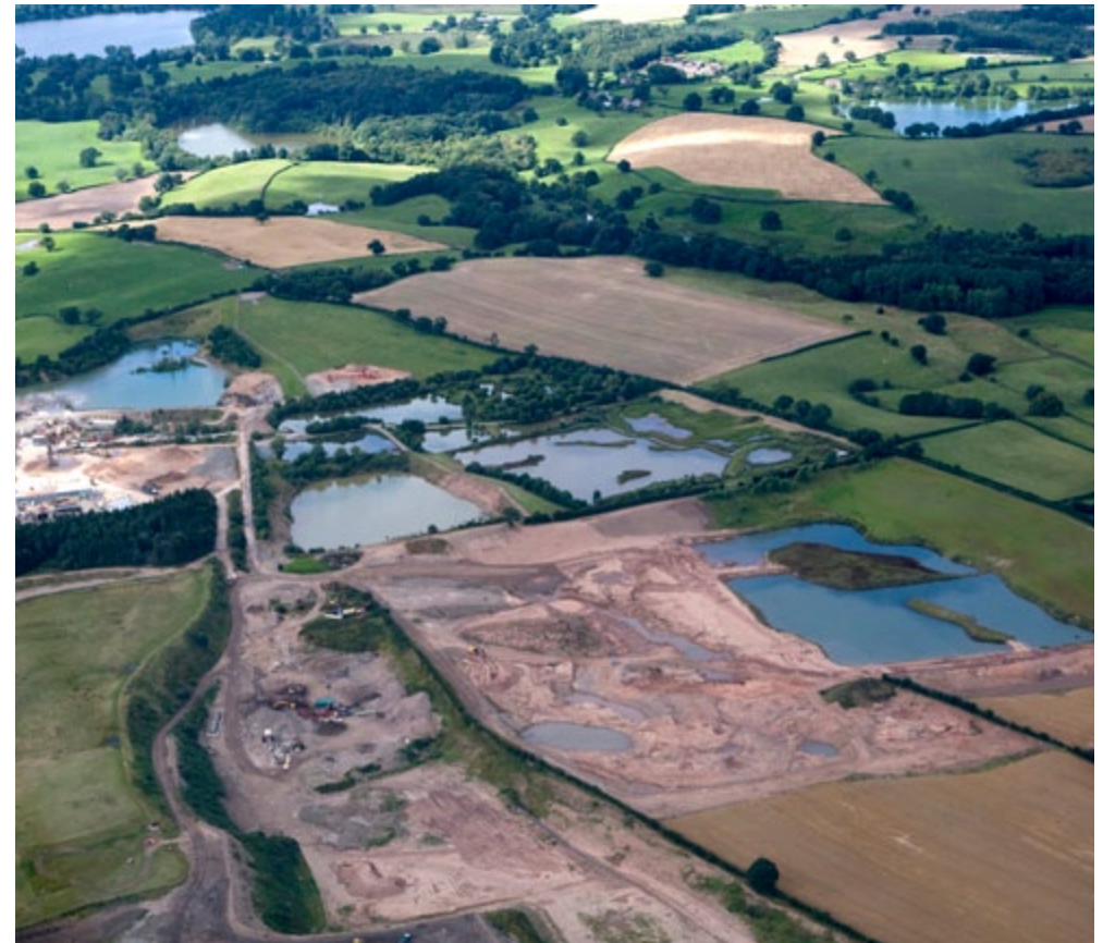
Active sand and gravel extraction at Wood Lane, just south of Ellesmere. As well as extracting economically important deposits of sand and gravel, the site also has landfill and waste recycling facilities. Working closely with Shropshire Wildlife Trust, the operator has also established part of the area as a nature reserve.
