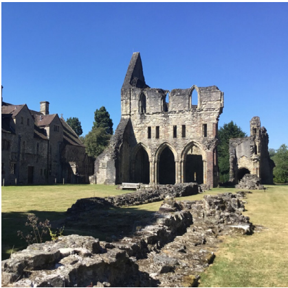
1. FROM WITHIN ST MILBURGA'S PRIORY LOOKING ACROSS THE GROUNDS
