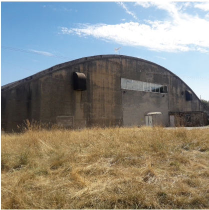
1. AN AIRFIELD HANGAR STANDS PROMINENTLY IN THE LANDSCAPE
