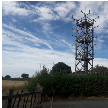
2. EARLY WARNING TOWER IS A PROMINENT DETRACTOR IN THE LANDSCAPE
