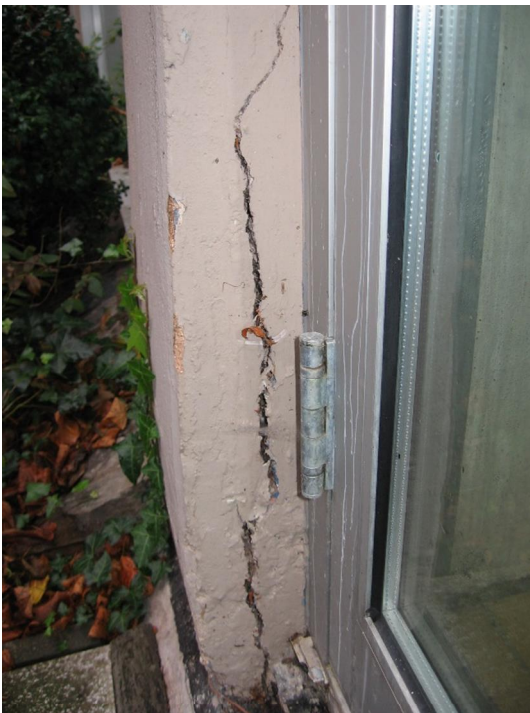
Figure 3 □ Vertical crack to concrete column on rear elevation
