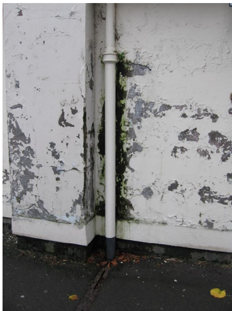
Figure 5 □ Façade damage caused by faulty rain water goods.
