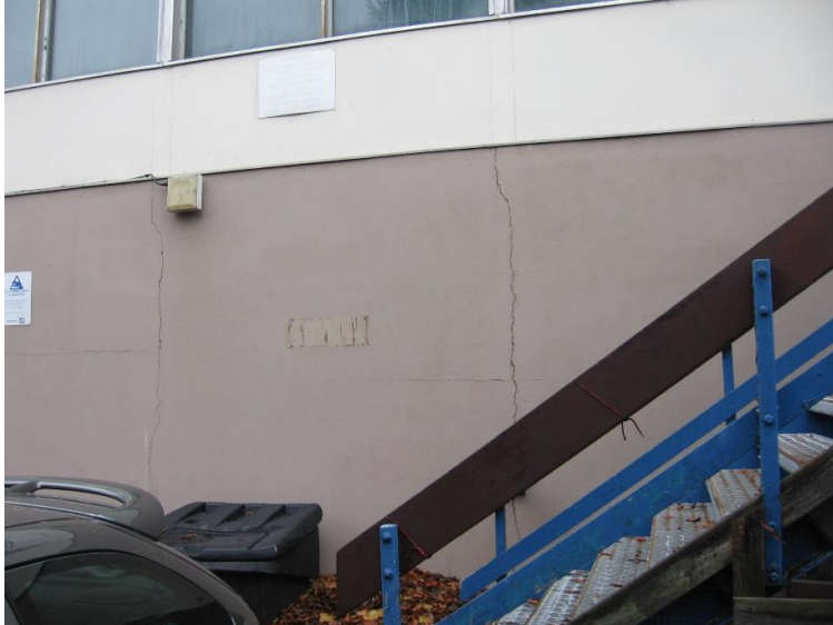
Figure 4 □ Vertical crack to concrete column on rear elevation
