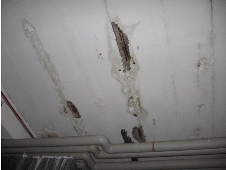
Figure 1 □ Spalling of concrete soffit as a result of reinforcement corrosion.
