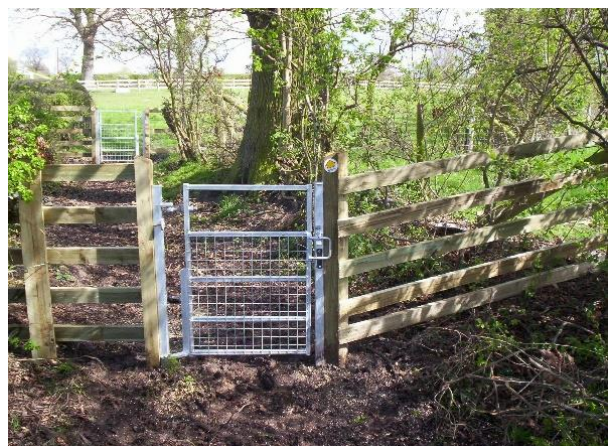
Figure 20- New Rights of Way gate installed
