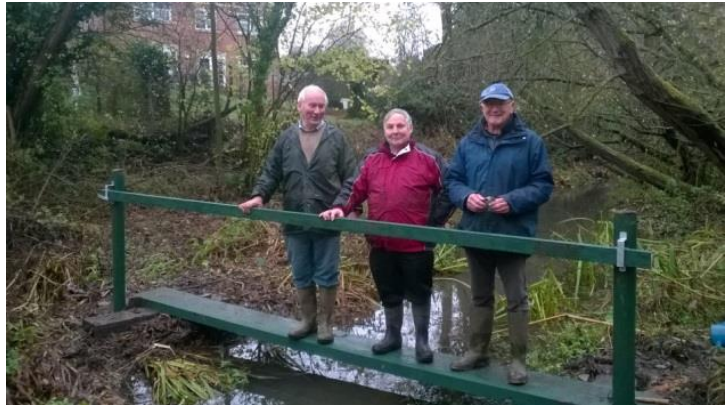
Figure 33- Installing a new bridge
