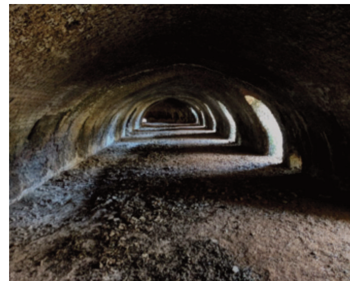
Figure 15 – Hoffamn Kiln, Llanymynech Limeworks – A Scheduled Ancient Monument
