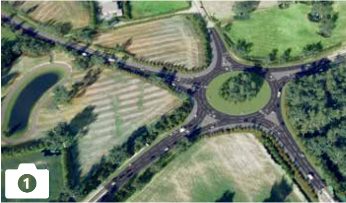
1 Drainage pond at Churncote roundabout (Camera facing east)
