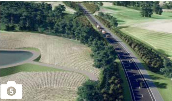
5 Berwick Road drainage pond (camera facing north east)
