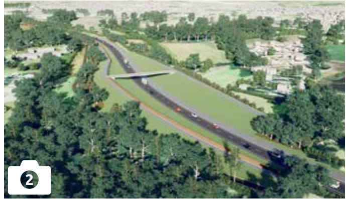
2 Cycle/footbridge and embankment east of Shepherds Lane (camera facing south east)
