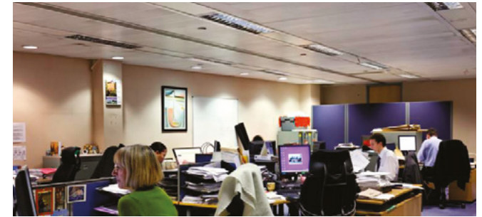
Figure 29: Poor UGR19 application
