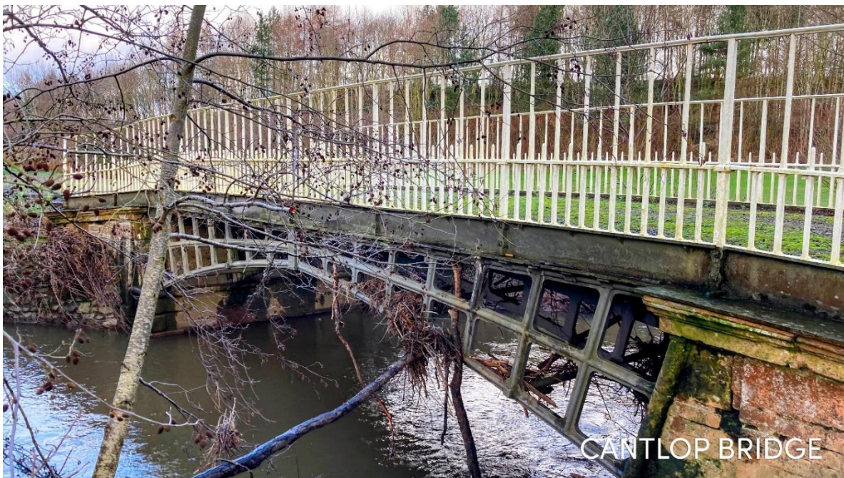
Figure 16: General View of Cantlop Bridge
