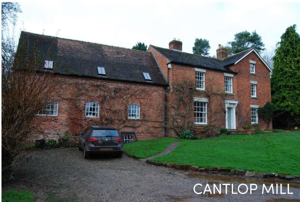
Figure 26: General View of Cantlop Mill
