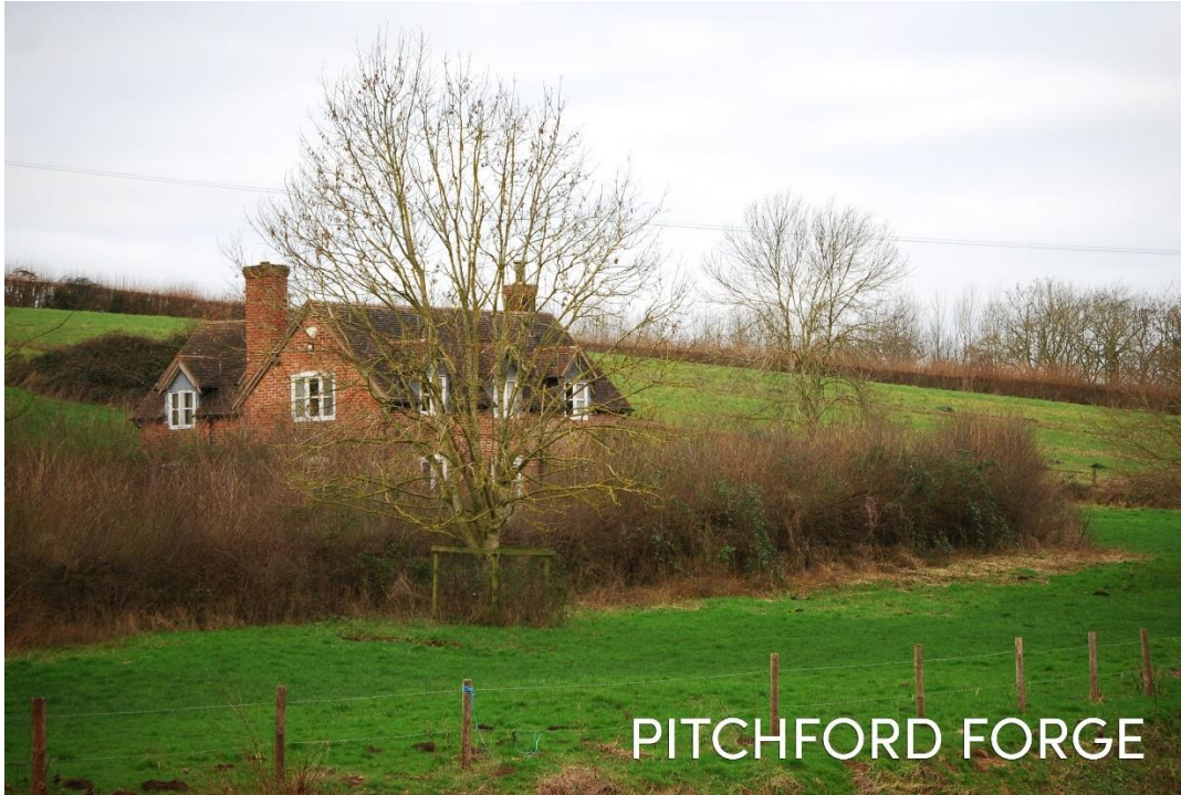
Figure 7: General View of Pitchford Forge
