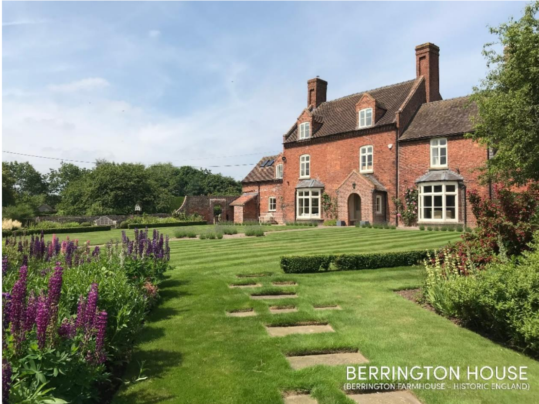
Figure 21: General View of Berrington Farm House
