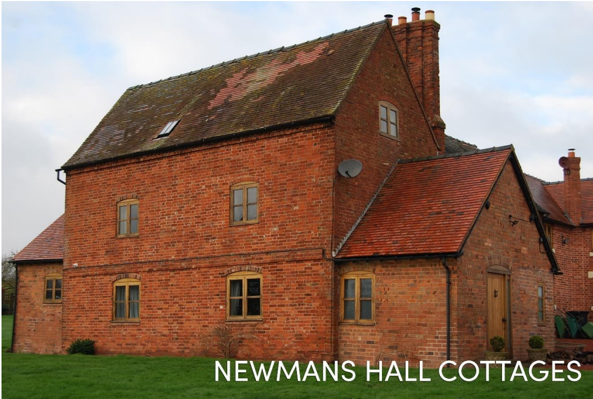
Figure 30: General View of Newman's Hall Cottages
