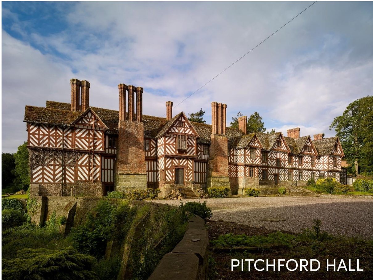
Figure 15: General View of Pitchford Hall
