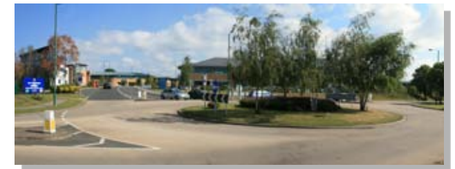
Shrewsbury Business Park (Phase 3) would be served from the existing Thieves Lane roundabout.
