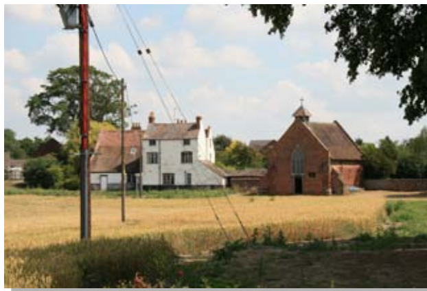
Older and more distinctive properties and individual buildings are located around the site and include the listed Sutton House and Sutton Church.
