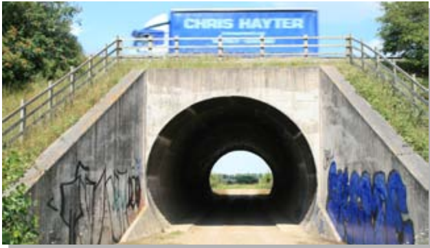
Existing A5(T) underpass in the south west corner of the site.
