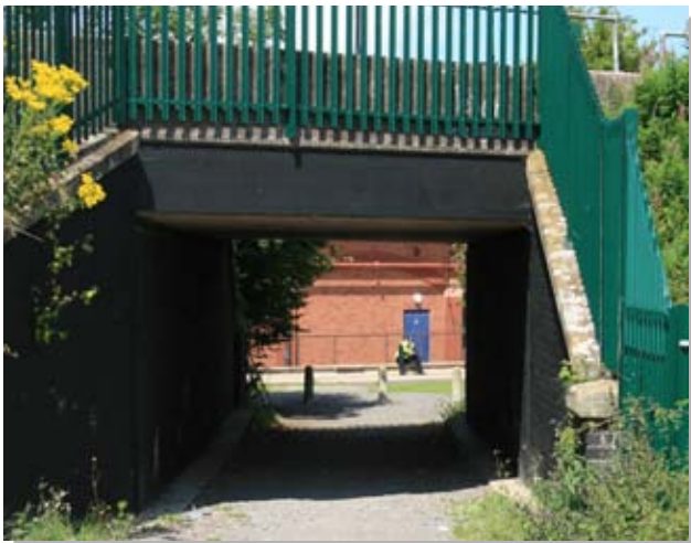
Existing rail underpass between the site and the Meole Brace Retail Park.
