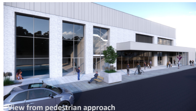
View from pedestrian approach
