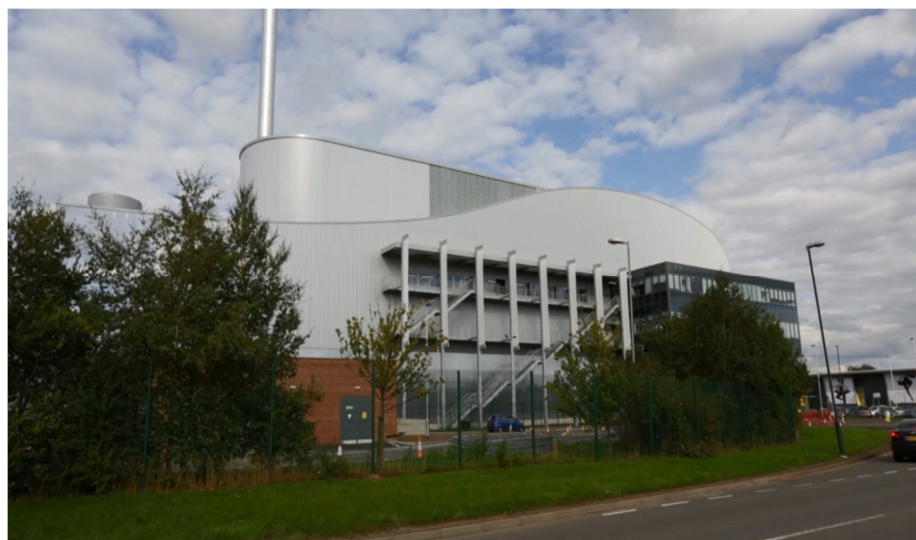
Figure 1 Veolia Energy Recovery Facility: Shrewsbury.
