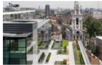
left examples of roof terraces and vantage points providing a unique experience and connection with the surroundings.
