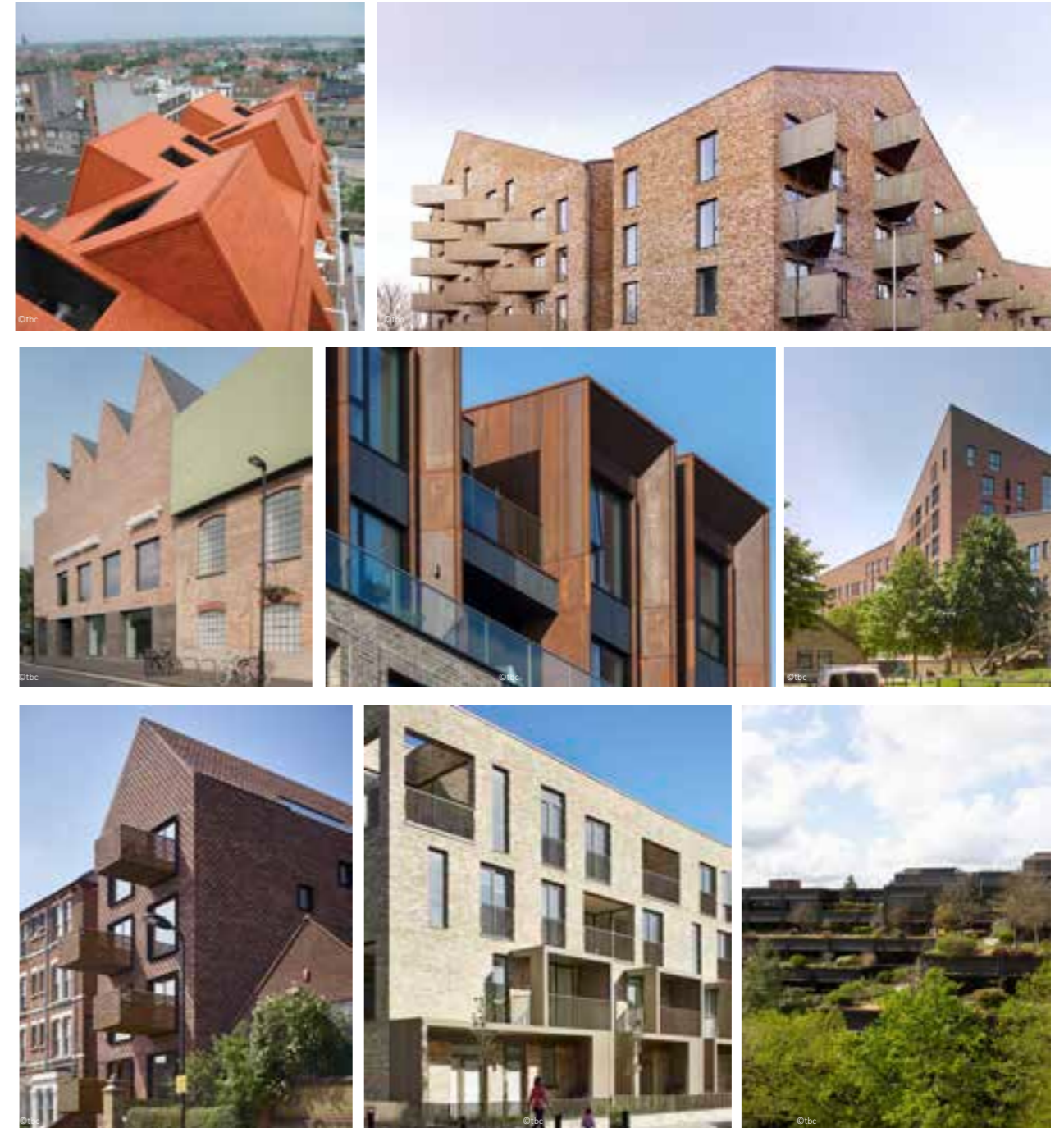
above visually interesting and contextual roofscape approach
