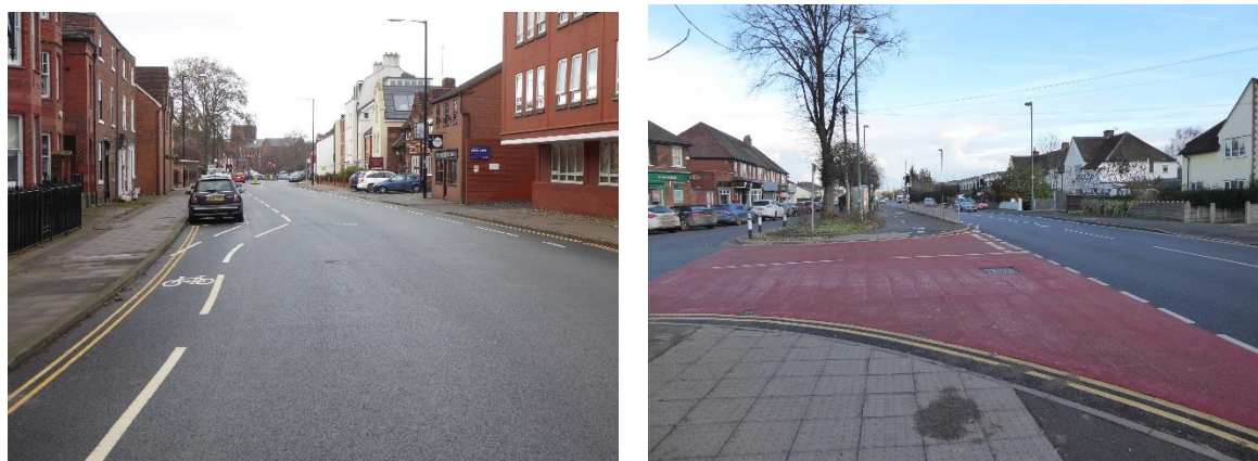
Figure 4. Recently delivered maintenance on Abbey Foregate, Shrewsbury (left) and Whitchurch Road, Shrewsbury (right)
