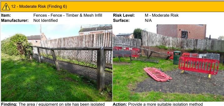
**Finding:** The area / equipment on site has been isolated from use however the area is still accessible and the means of isolation has either introduced additional hazards that may cause harm in the event of users accessing the area or is insufficient to stop users from accessing the equipment
