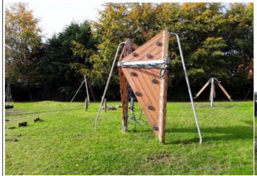
**Finding:** This item of equipment has a fall height in excess of 2.5m and grass mats have been installed as an impact absorbing surface; these mats rely heavily on the underlying surface to achieve their critical fall height properties.
