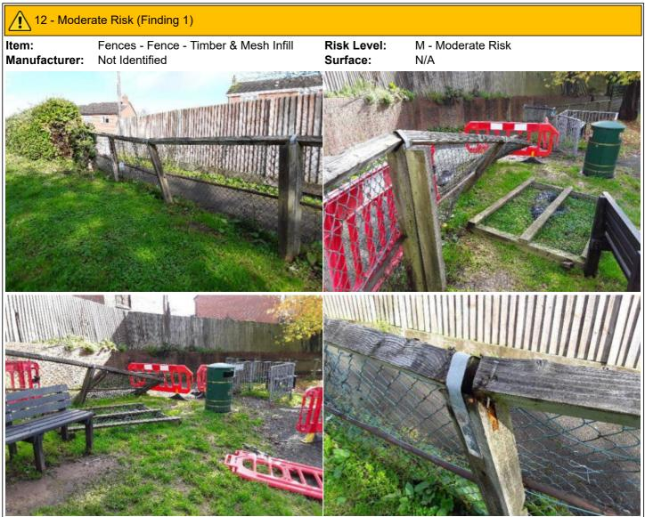
**Finding:** The fence has severe rot and is damaged exposing projecting fixings and there are unsecured sections of fencing within the play area
