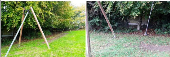
**Finding:** The seat is less than 2.0 metres from the post when extended at 45 degrees at the end of the area of travel minimum distance is maintained and does not meet the requirements of BS EN 1176 Part 4
