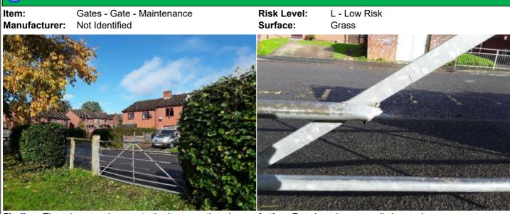
**Finding:** There is some damage to the item creating sharp **Action:** Repair and remove all sharp edges edges
