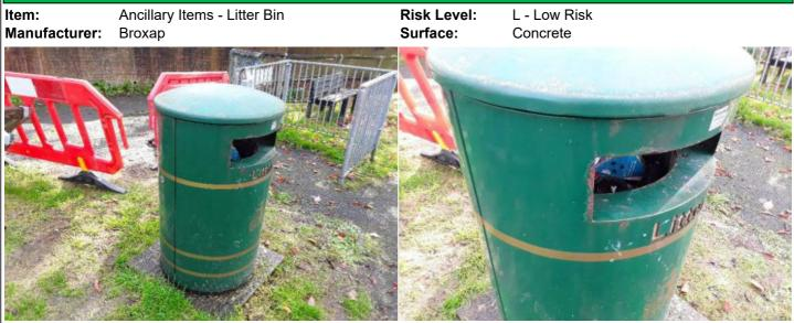
Finding: The paintwork on this item has been damaged or Action: Treat affected areas and repaint worn exposing the metal underneath which is rusting / corroding
