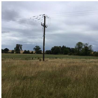
4. FROM PROW, VIEW NORTH EAST
