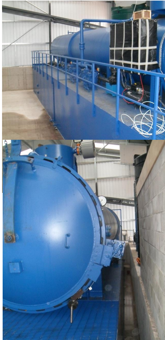
Figure 3: Tanalith E Plant 1 during installation
