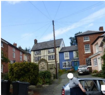
Telegraph pole on the Square – Zone 2
