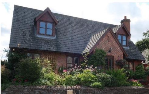
Dormer windows and front portico Zone 7
