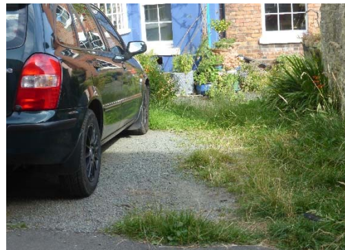
Weeds growing in the perimeter access track.
