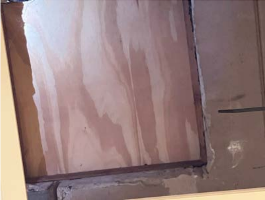
Photograph 6 unsupported openings filled with plywood.
