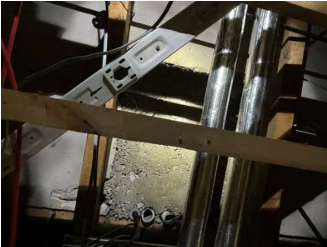
Photograph 16 cut panel infilled with concrete and supported on timber joists.
