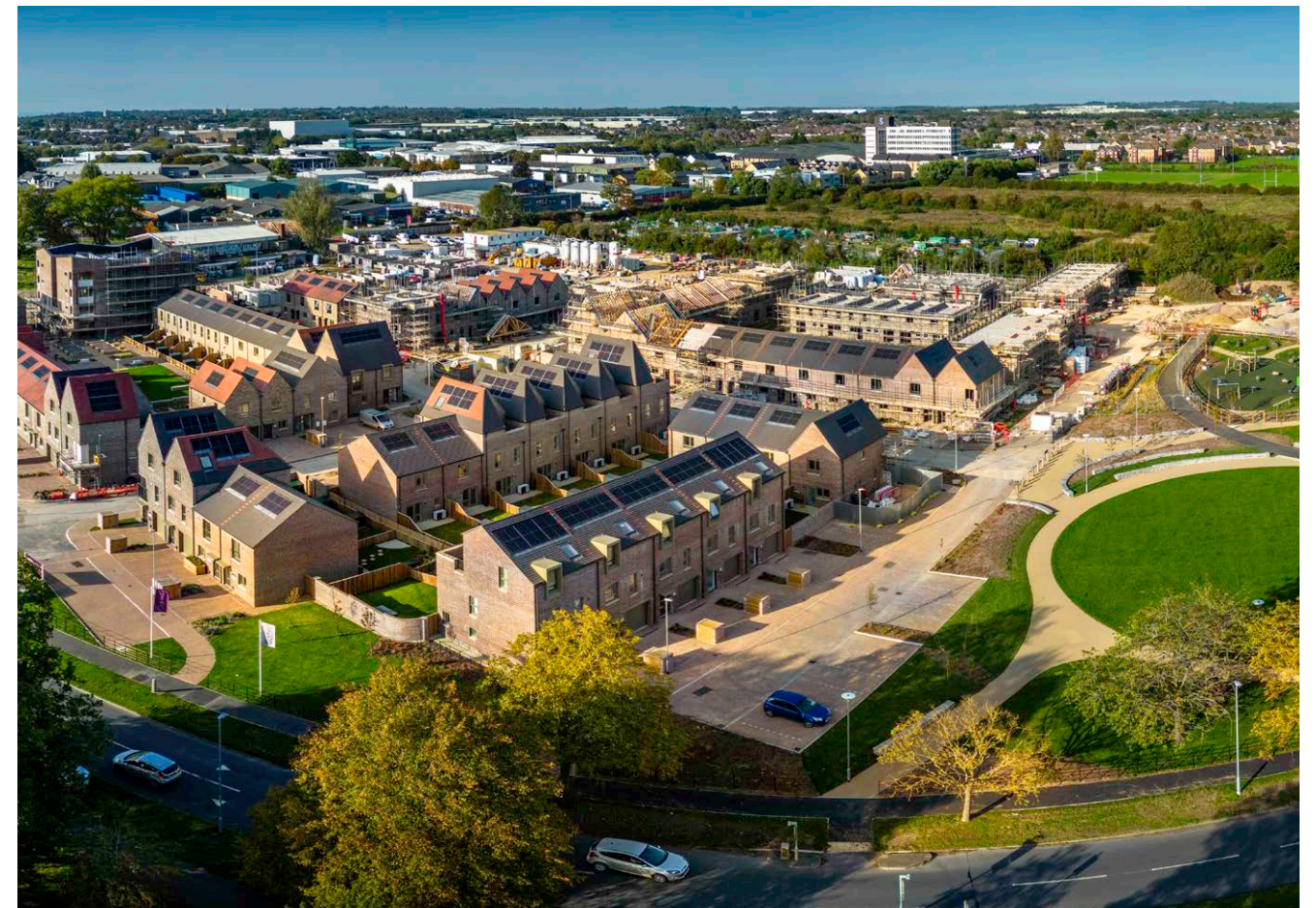
Examples of Lovell sites under construction
