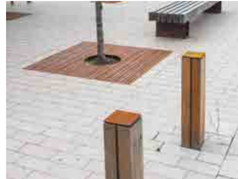
Timber bollard with corten top
