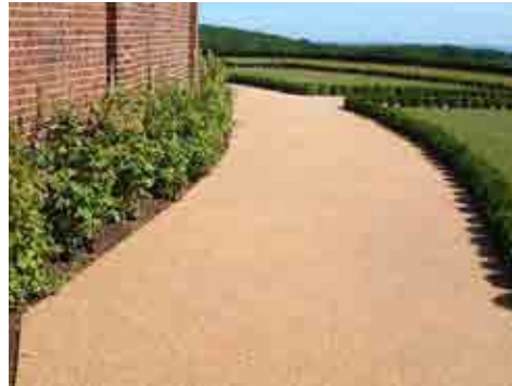
Resin bound gravel - Restricted to the eastern end of the development proposals
