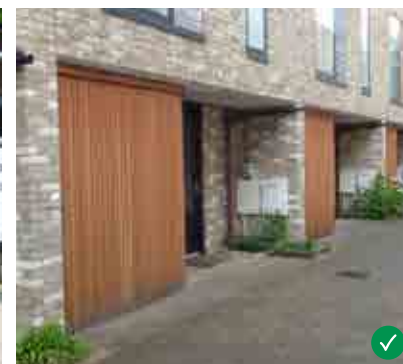
Utility meters mounted on oblique facing wall with provision of landscape planter for additional screening
