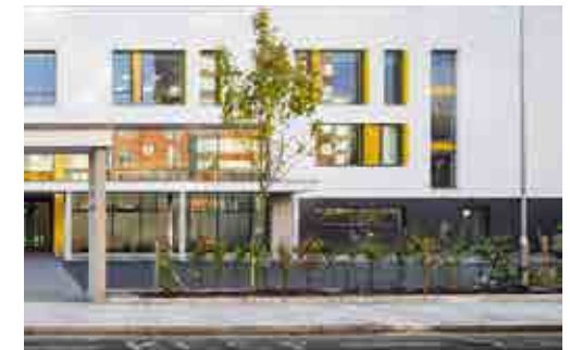
School boundary to be clearly marked and defensible while allowing inter visibility
