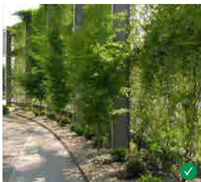
Examples of well integrated planting strategies can be used for proposed pumping station and substation
