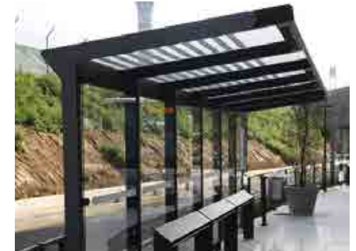
Bus shelter with perch seating
