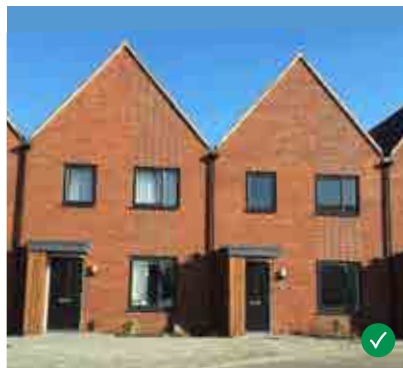
Rainwater pipes breaks facade into 'individual modules' and reflect rhythm.
