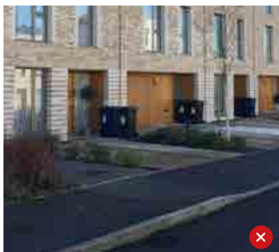
No provision for refuse bin detracts from the overall quality and appearance of the buildings
