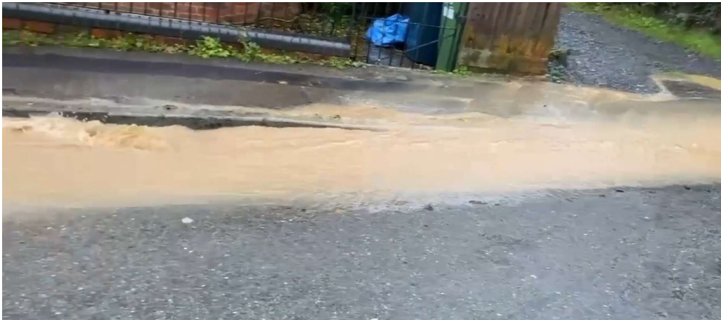
Photos 13-16 Showing Lyth Hill Road October 2023
