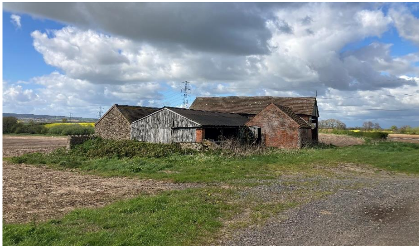
Traditional farm buildings, Near to Horn Cottage
