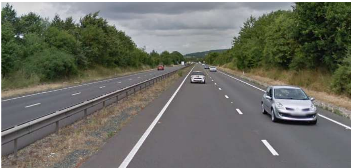
Photograph 2.5 : A5 – Westbound (source: Google Maps)
