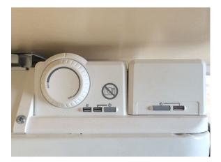
The electric wall heater is operated by pressing the on/off button followed by the boost button. The controls have been set to approximately 25 degrees; there will be no greater heat output from the heaters even though the dial still moves. If your room is particularly cold, there is a Boost button, which will provide full heater output for a two-hour period.
