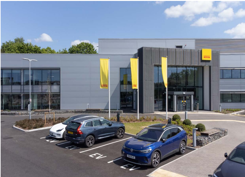
Sandvik | Halesowen | Completed Building
